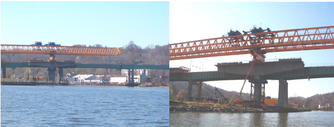
Gantry for Roslyn Viaduct construction.
